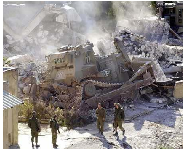
[illustration 12] D-9 Bulldozer demolishes Gaza's radio station
